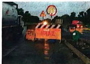
The work is ongoing on a 121-km stretch of NH-48
